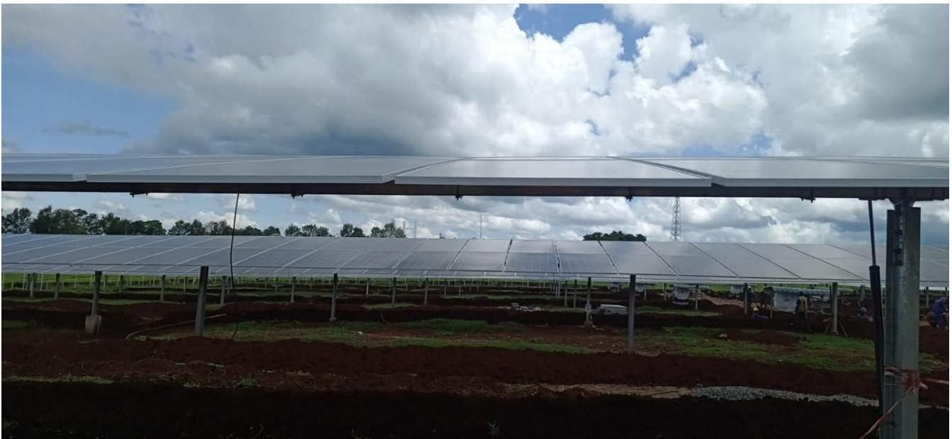
Figure 3; Solar Installations & Structural Footing
